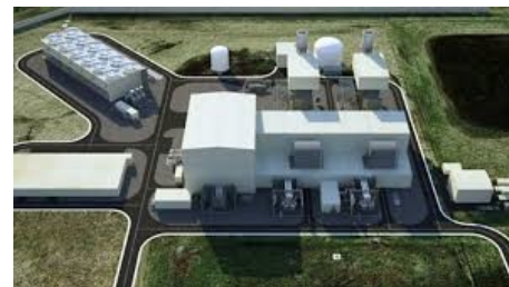
St. Joseph Energy Center
